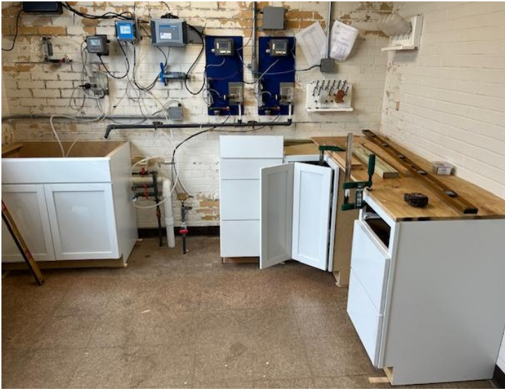
Lab renovation at plant 1
