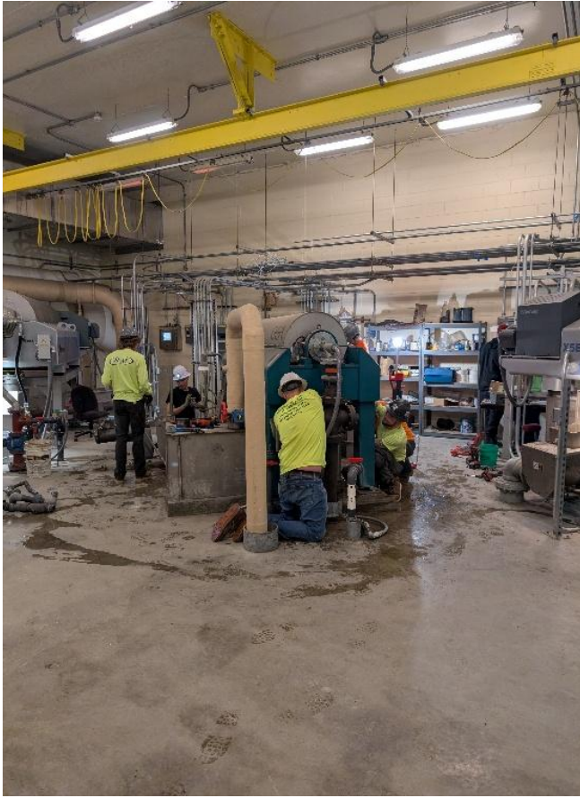
Old Centrifuge #1 Tear Down
