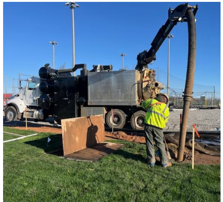
New conduit being installed to well 9
