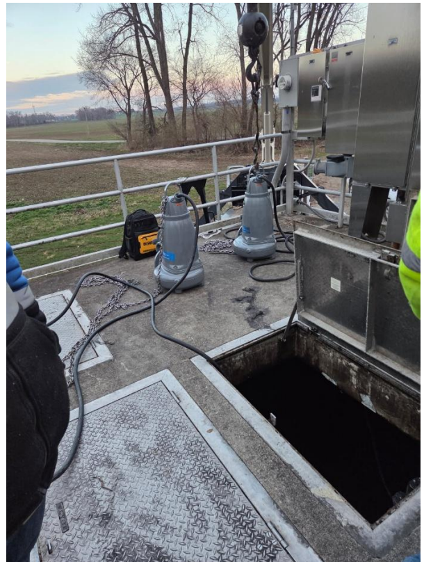
Two Pumps Put in for 8 th Street Lift Station
